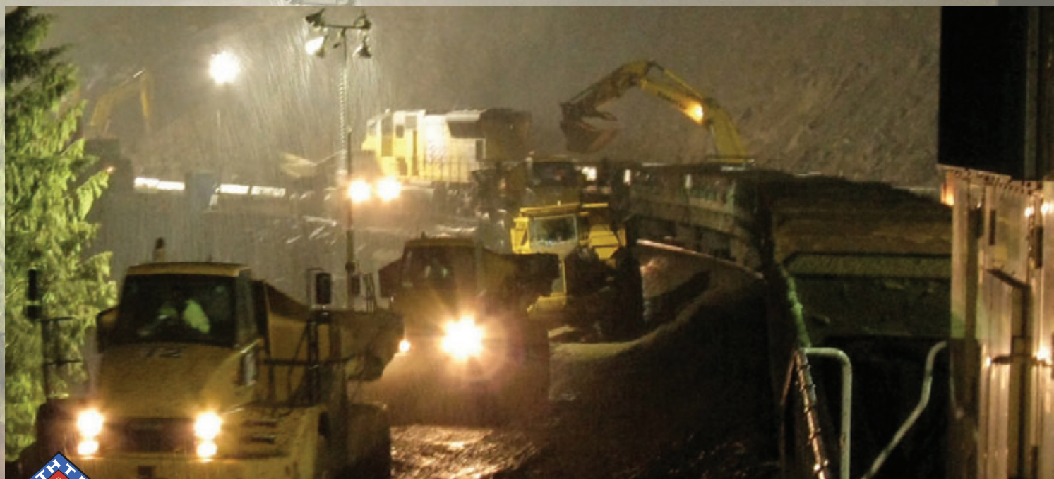
Night operations on the Frazier Slide
