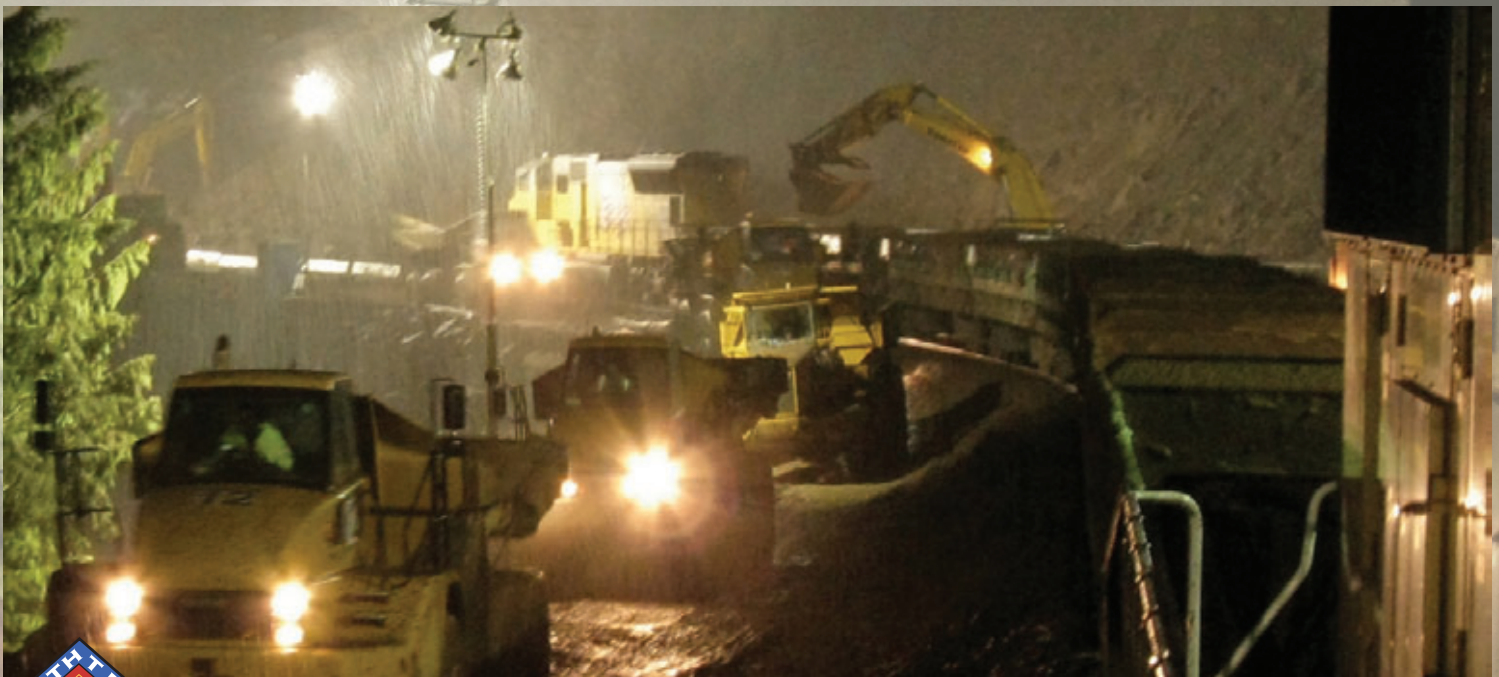
Night operations on the Frazier Slide
